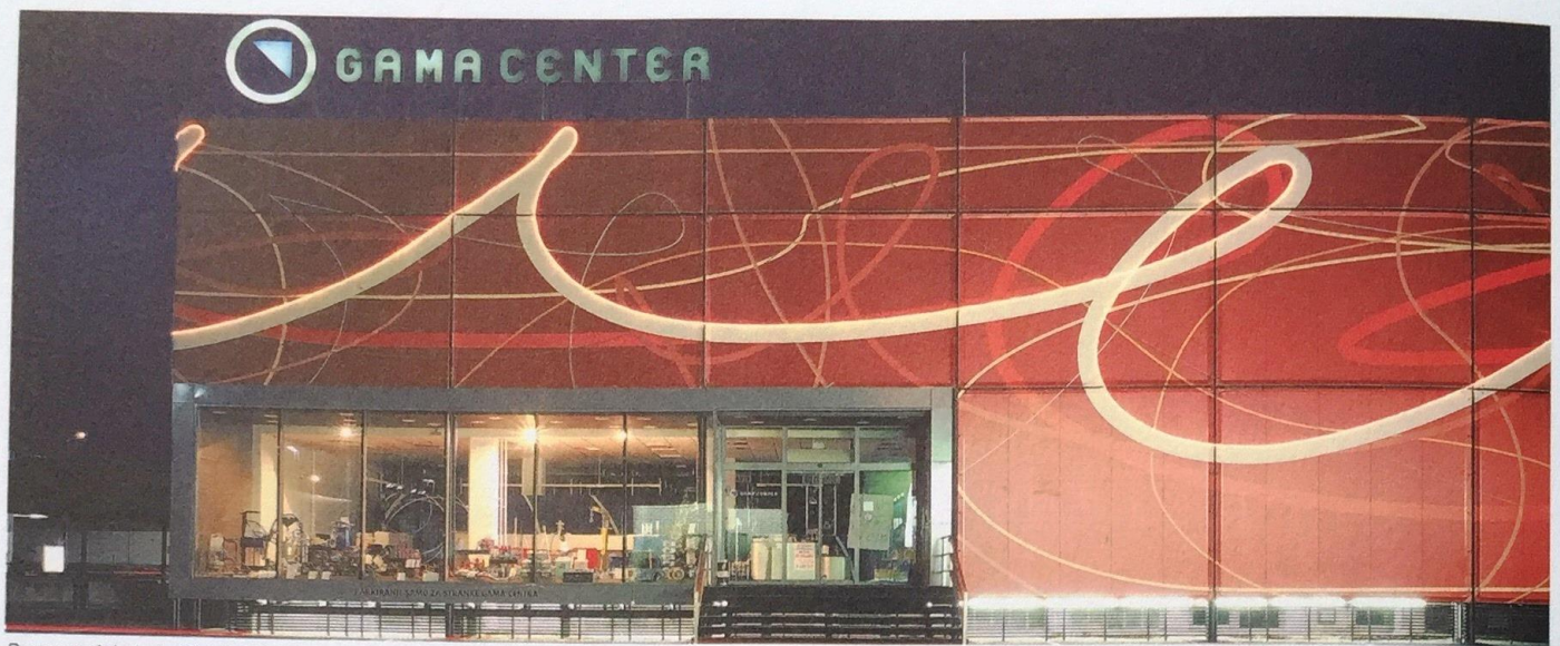
Prenova dela hale 10 v BTC-ju, trgovina Ariel in Gama center
